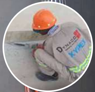
Treatment of Joint Detail using Xypex
