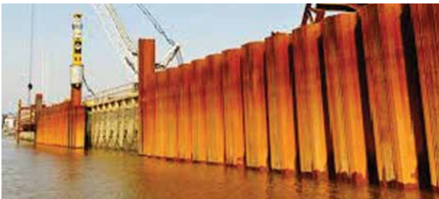
Sheet piles application at coastal areas
