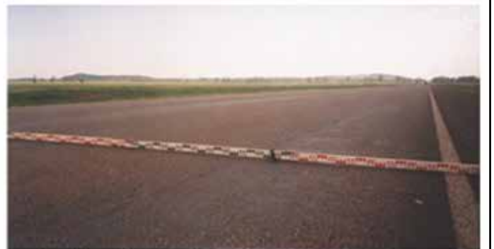
Road section today
