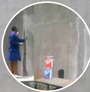
Crack repairs on a water tank using Xypex
