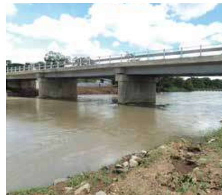
Aswa Bridge (Completed)
