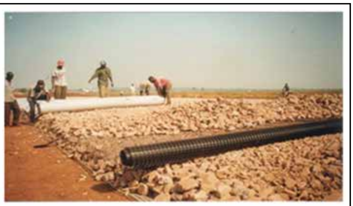
rolling geotextile and geogrids to Form filter
