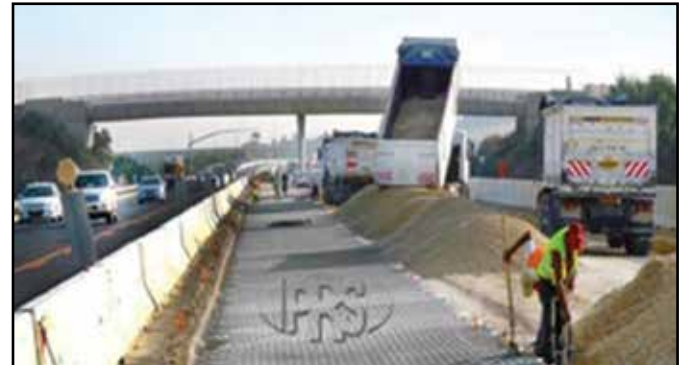
Layer of geocells prepared
