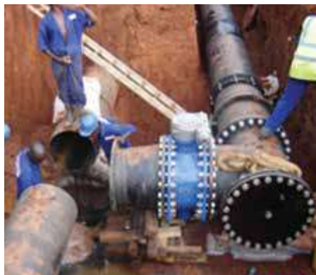
Kampala Water and Sanitation Programme Phase 1 – Component 3 Transmission Mains (completed)
