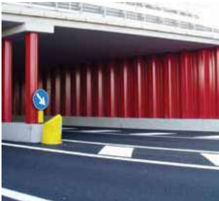
Sheet piles for bridge abutments
