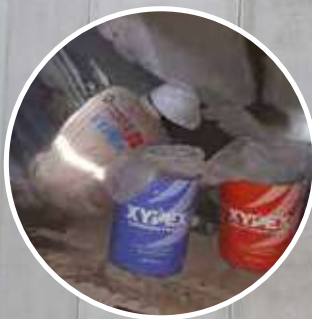
Crack repairs in a dam using Xypex
