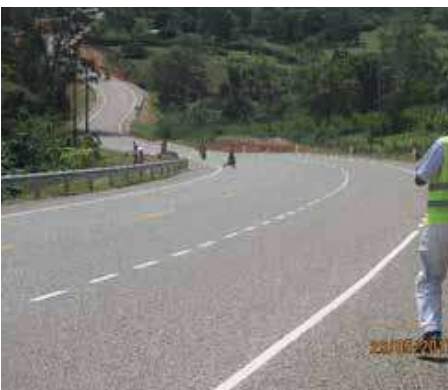
Consultancy services for construction supervision for the upgrading of Kamwenge – Fort Portal Road 66.2 Km (completed)
