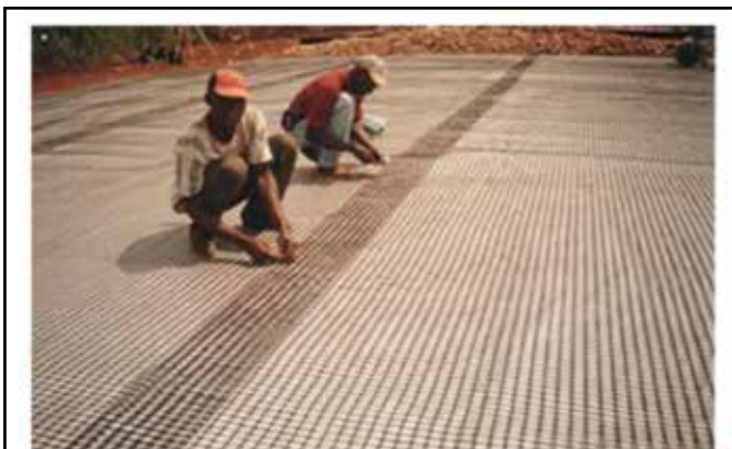
Tying geogrid overlaps at subgrade
