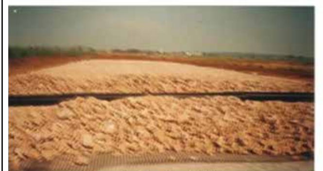
Stone filter before backfilling
