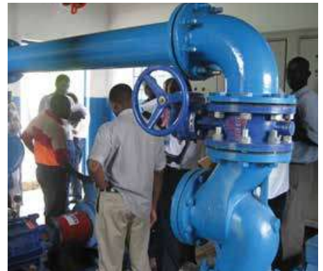
Gulu water supply and sanitation project (completed)
