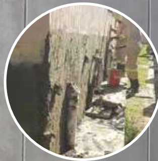
Treatment of rising damp using Xypex
