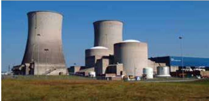
Figure 2: The TVA nuclear power plant in the US
