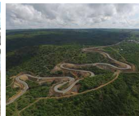
Kingfisher access roads in the Albertine area 17 Km (completed)
