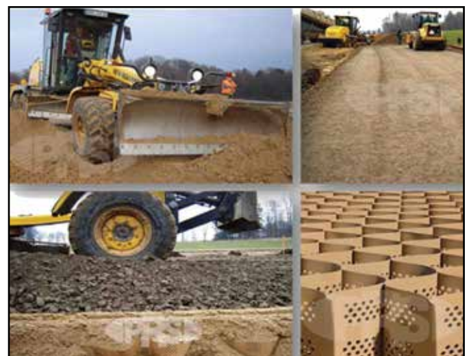
Illustration of the procedures of Geocell Installation
