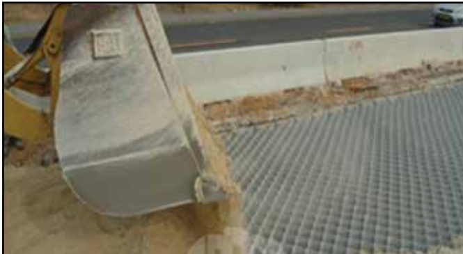
Infill of materials into the Geocells
